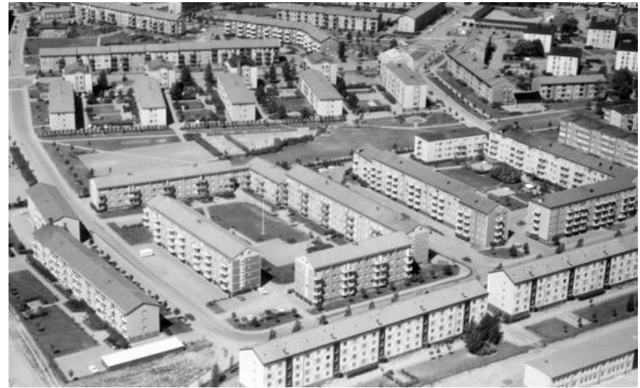
Renovation, Salabackar, Uppsalahem Phase 1 – change of windows
