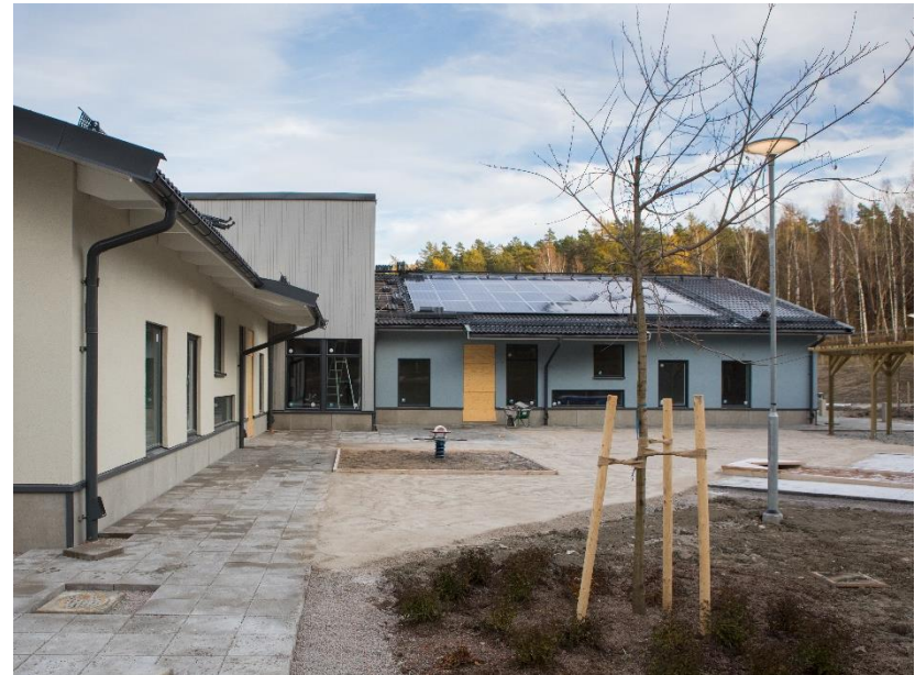
Construction, Arboga kommun, Social properties, i.e.
